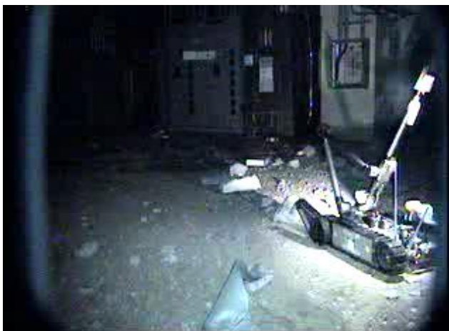
Robot advancing on the first floor of the Unit 1 reactor building (April 17, photo provided by TEPCO)
